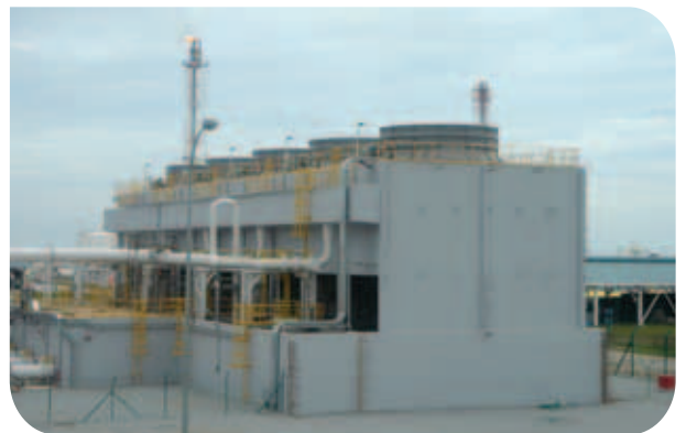
:: Malacca Cogen Power Plant, 12,500 m 3 /hr (5 cells).
